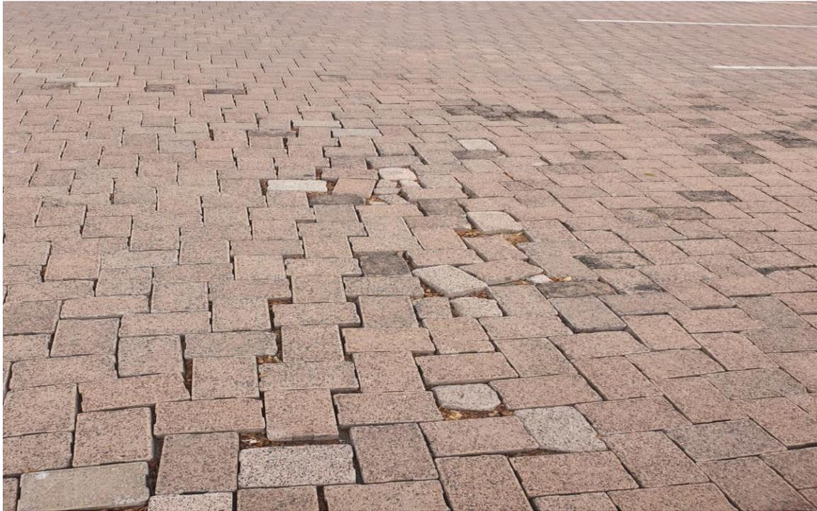
*Figure A-3: Wits Upper Parking indicating poor construction/maintenance resulting in failure of the PPS.*
