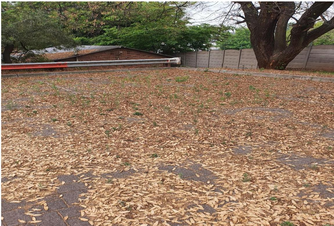
*Figure A-2: Wits Upper Parking indicating clogging and blockage of the PPS*
