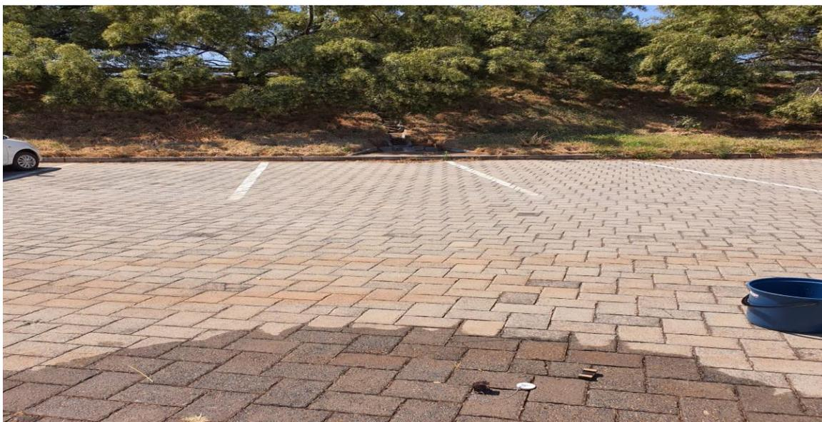
Figure 3-3: Wits Parking Paving Type – similar type used for both upper and lower parking lots.
