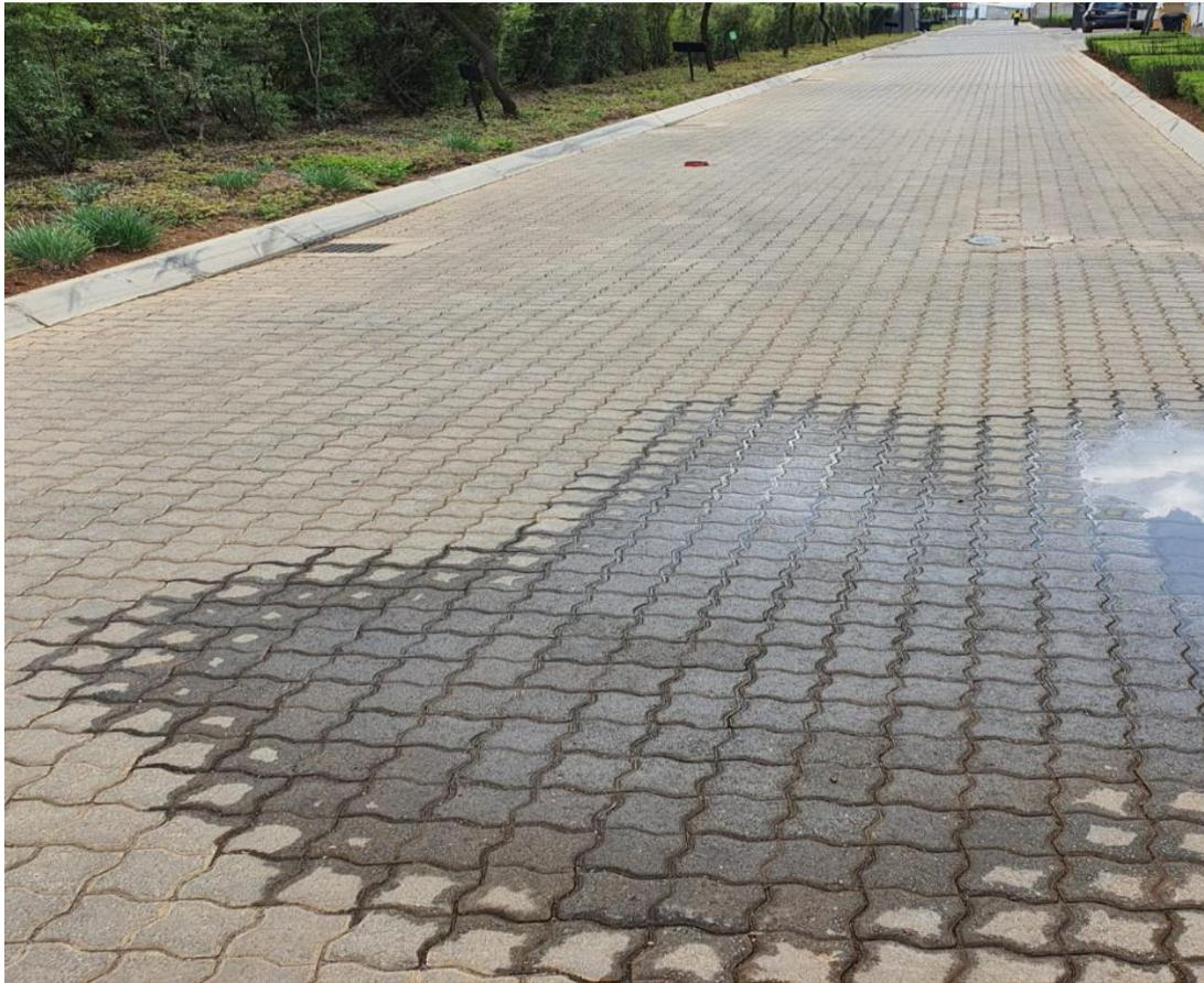
*Figure 3-6: Toyota Type 1 - also indicating slope towards multiple drainage points*
