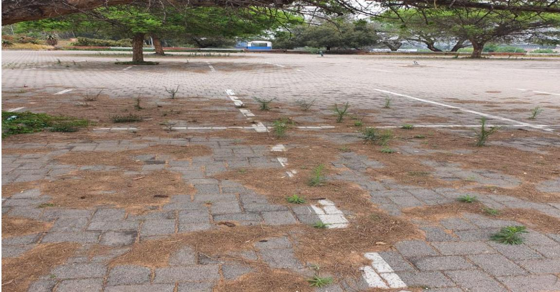
*Figure A-1: Wits Lower Parking indicating clogging of the PPS..*
